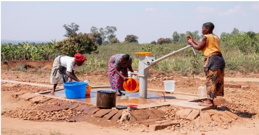
Photo 1: A Borehole fitted with an Afridev hand pump (a community-based management technology)
